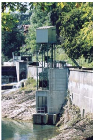
Fischlift, Birs (Hydrosolar)
